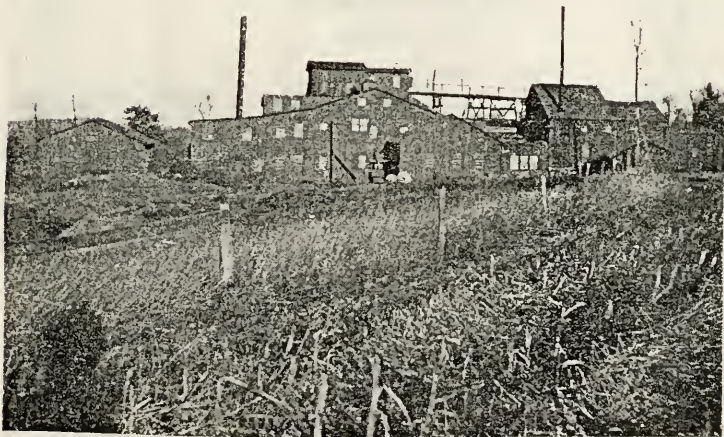
Fig. 98 View of another graphite mill near Byers. •Note the large scale, frame construction. It did not survive long after the mills were closed. In many cases the lumber was salvaged, and the plants slowly disappeared into the surrounding fields. Benjamin Miller, Topographic and Geologic Survey of Pennsylvania Report #6: Graphite Deposits of Pennsylvania (Harrisburg, PA: C.E. Augenbaugh, PA State Printer, 1912), plate XI.
